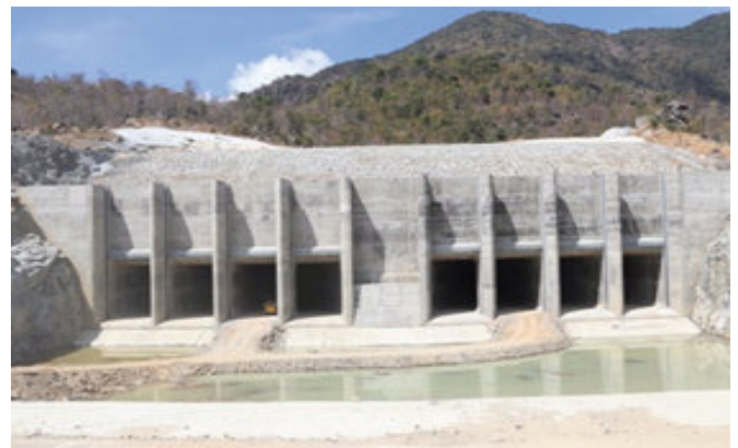
Outlet works completed in March, 2021
