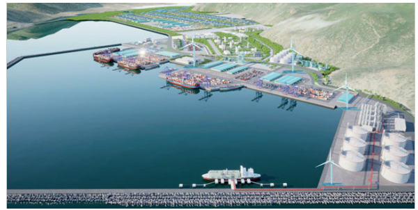
Ca Na Green Energy Complex (Ninh Thuan)
