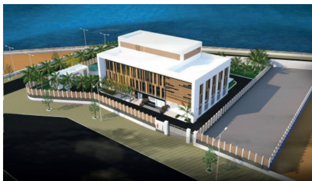
Overall of Hai Chau 220kV Substation (Front)
