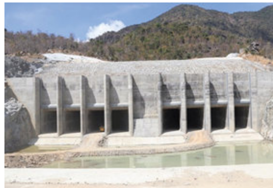
Outlet works completed in March, 2021
