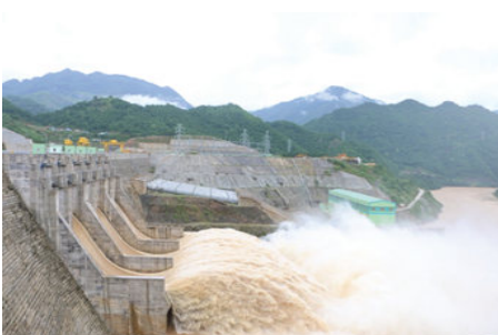
Trung Son Hydropower's dam spillway
